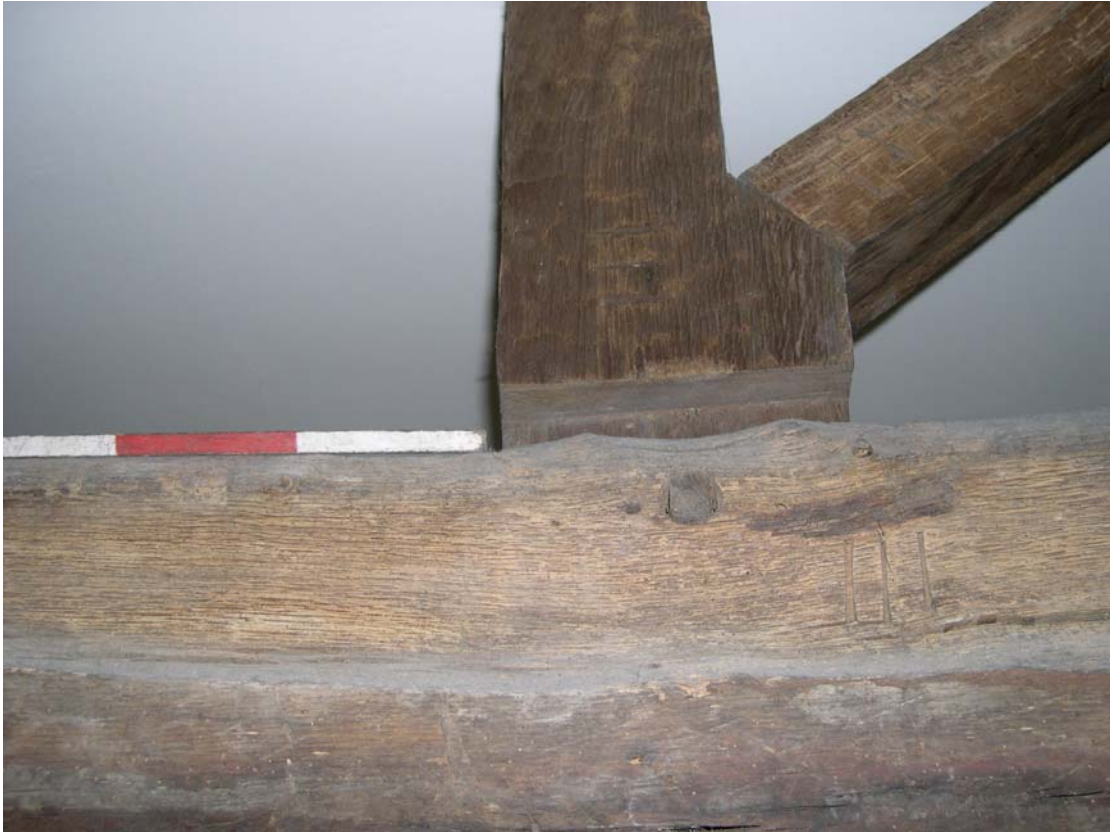
Plate 16: Assembly marks on farmhouse truss
