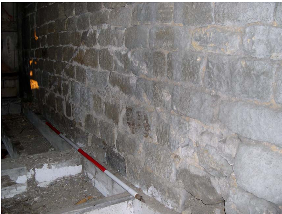
Plate 41: Roof-line scar in northern attached cow-house
