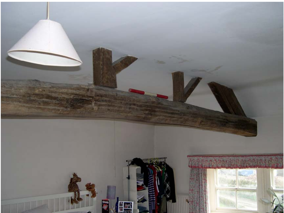
Plate 15: Queen and princess posts in farmhouse truss
