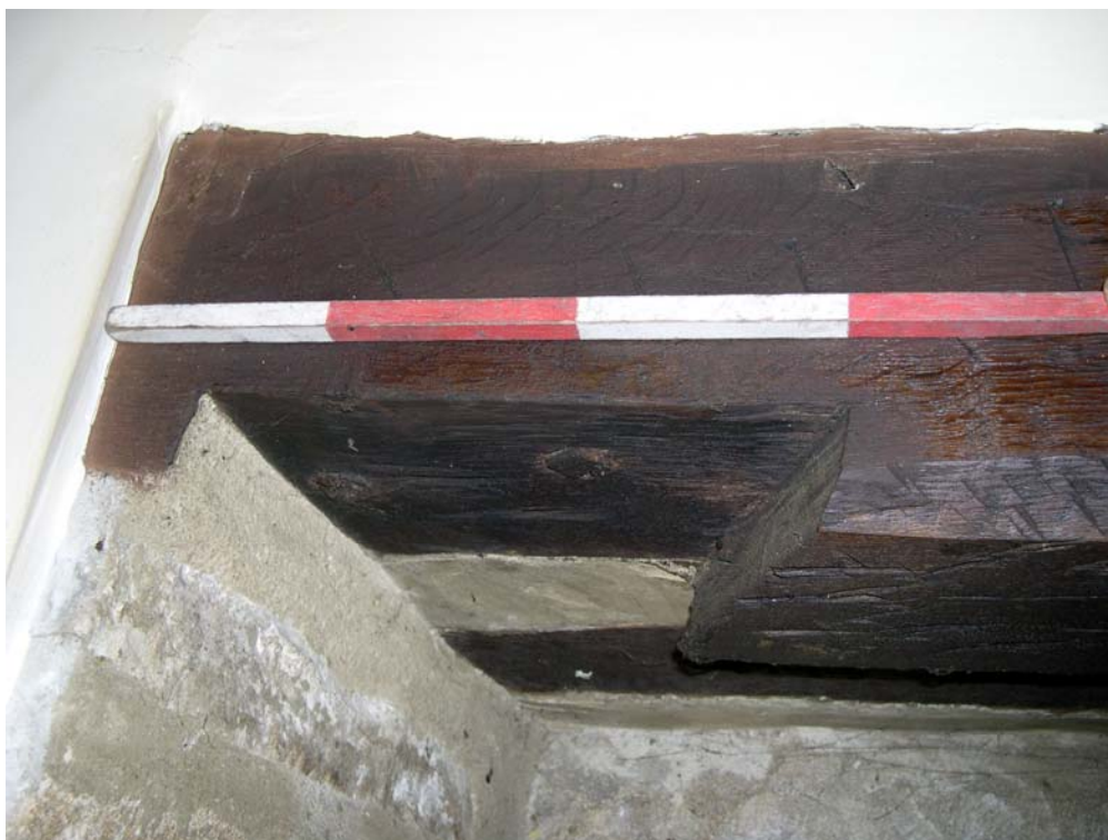
Plate 11: Re-used lintel above farmhouse door
