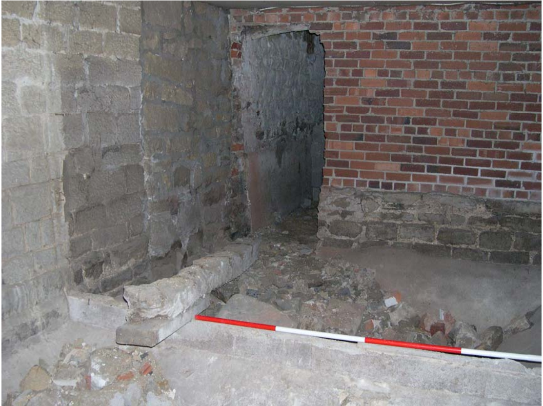
Plate 34: Eastern bay of the barn, showing phased stonework
