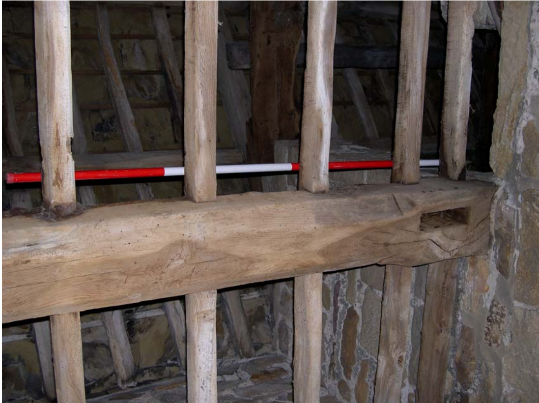
Plate 30: Mortice within re-used beam in the barn porch
