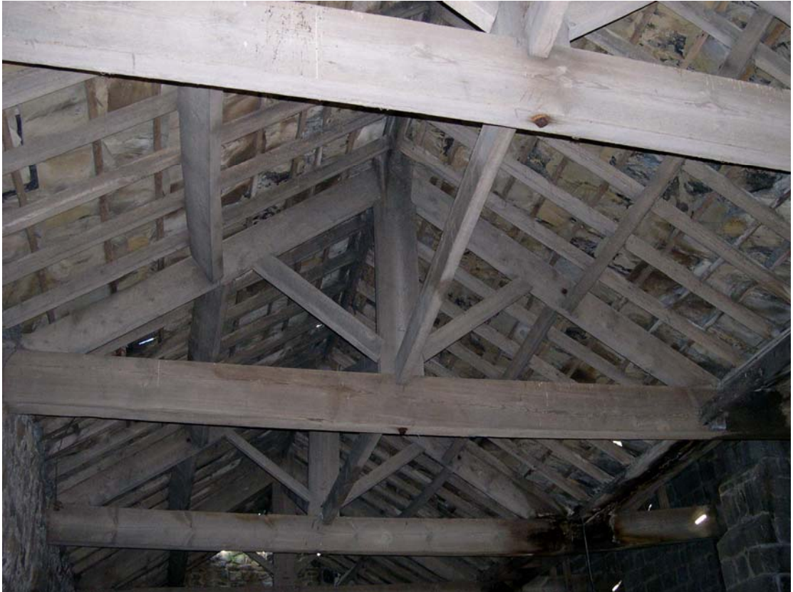
Plate 44: Roof trusses in attached cow-houses
