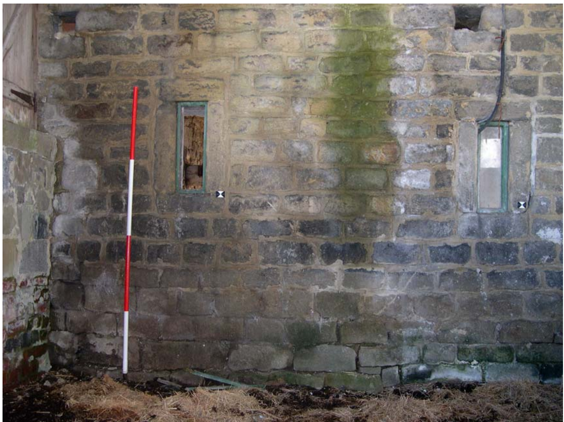
Plate 25: Glazed vents in north elevation of the cow-house
